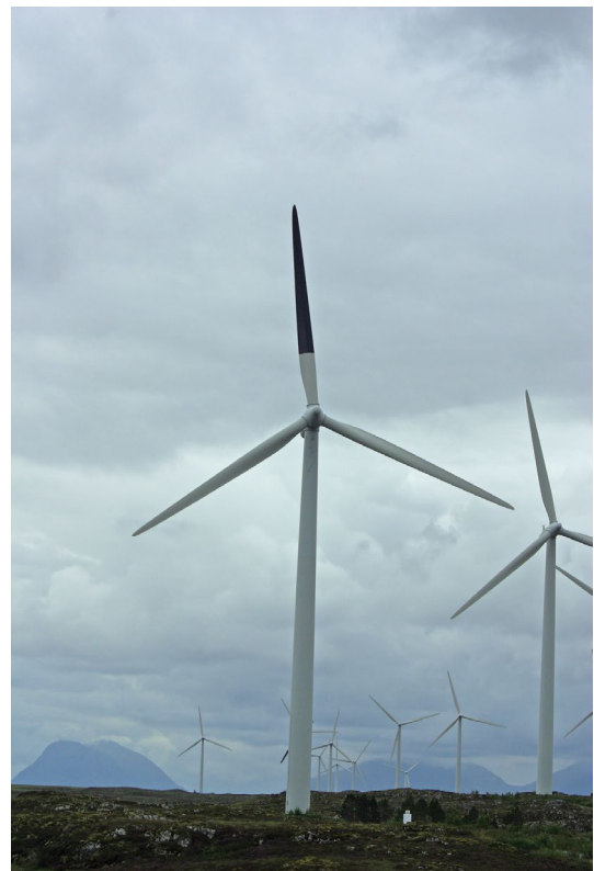
FIGURE 1 Wind turbine in the Smøla wind-power plant with painted rotor blade
